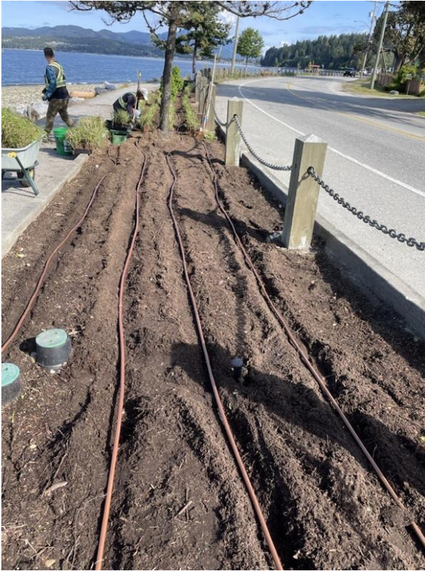
Drip irrigation added to a garden bed
