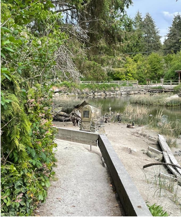
Before: Landscape ties lifting off rebar with high tides
