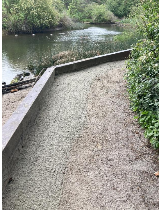
After: landscape ties secured and aggregate added to walking path
