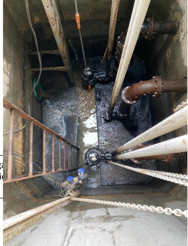
Mackenzie Lift Station, before and after annual clean. Note significant grease on the surface.
