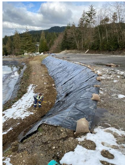
Repurposing an old liner to prevent vegetation growth at the Dusty Road site.
