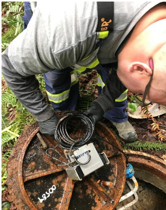
Portable monitoring device installed in the collection system.
