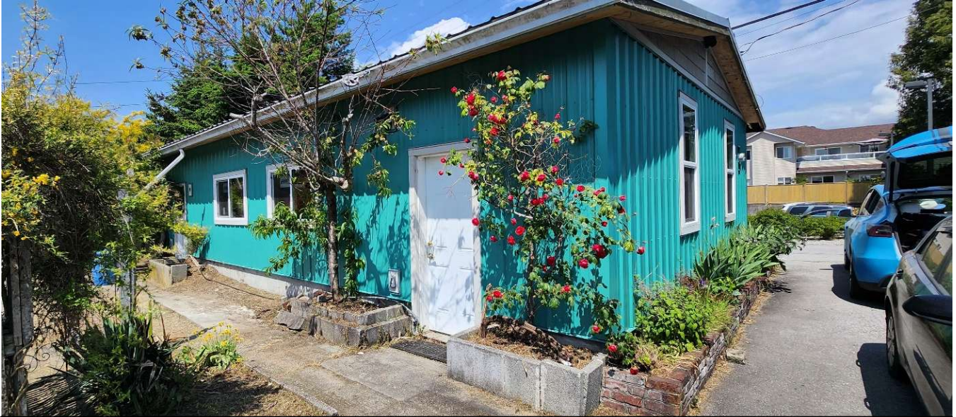
Photo – south and east facades of existing garage building.
