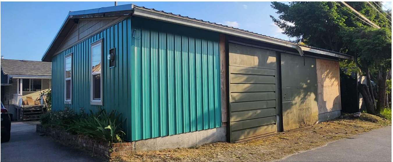
Photo – north and east facades of existing garage building.
