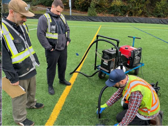
Staff learning the process to repair artificial turf.
