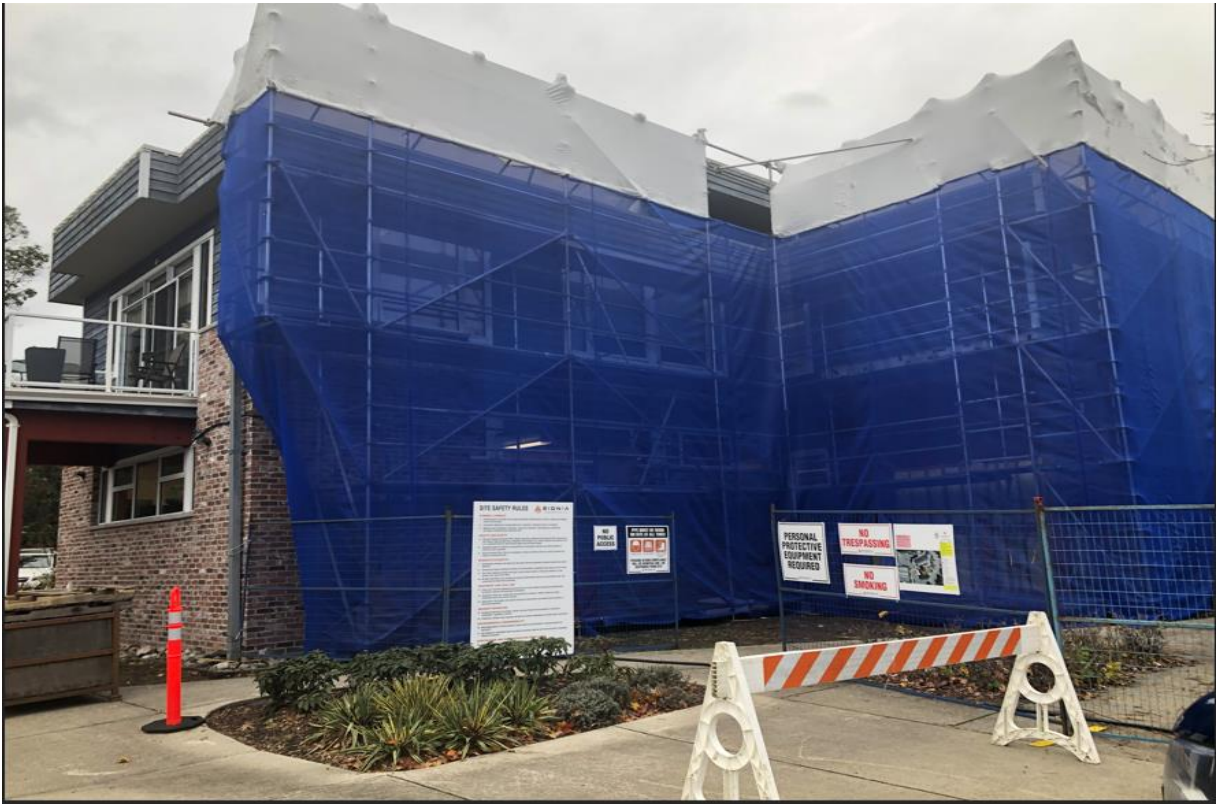
Photo of the Municipal Hall and Library Remediation
