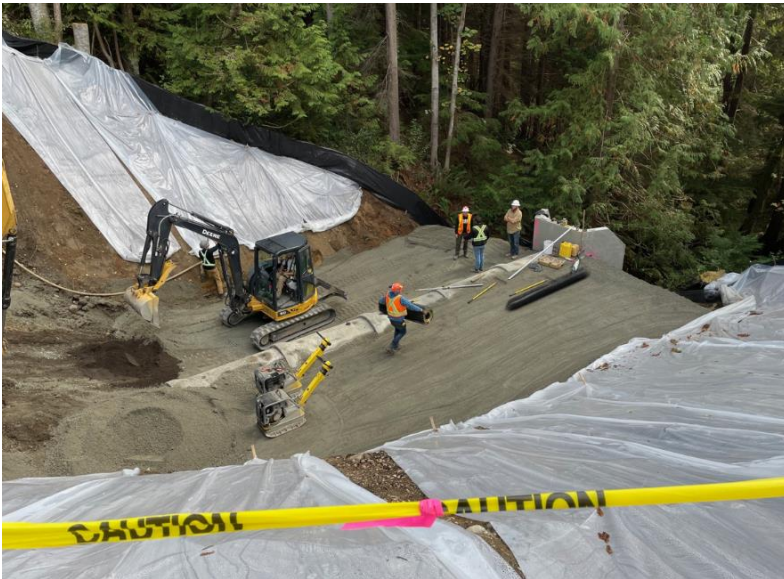
Wakefield Road Culvert- Pipe Installation
