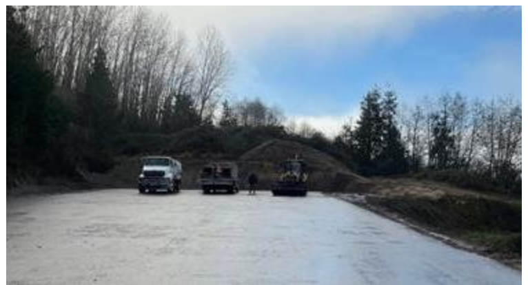
Site after removal of septage solids.
