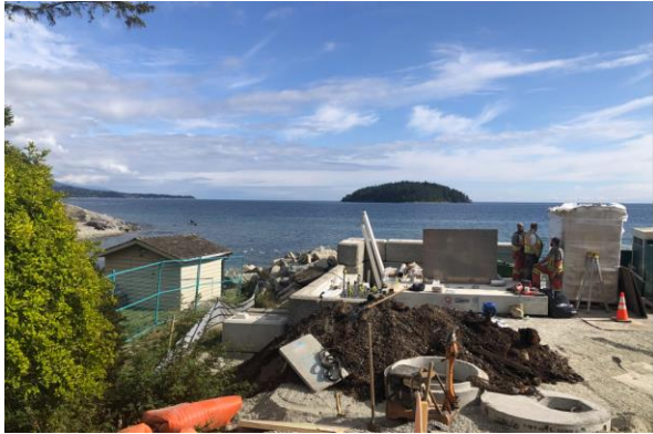
Wakefield Lift Station-Wet well lid installation
