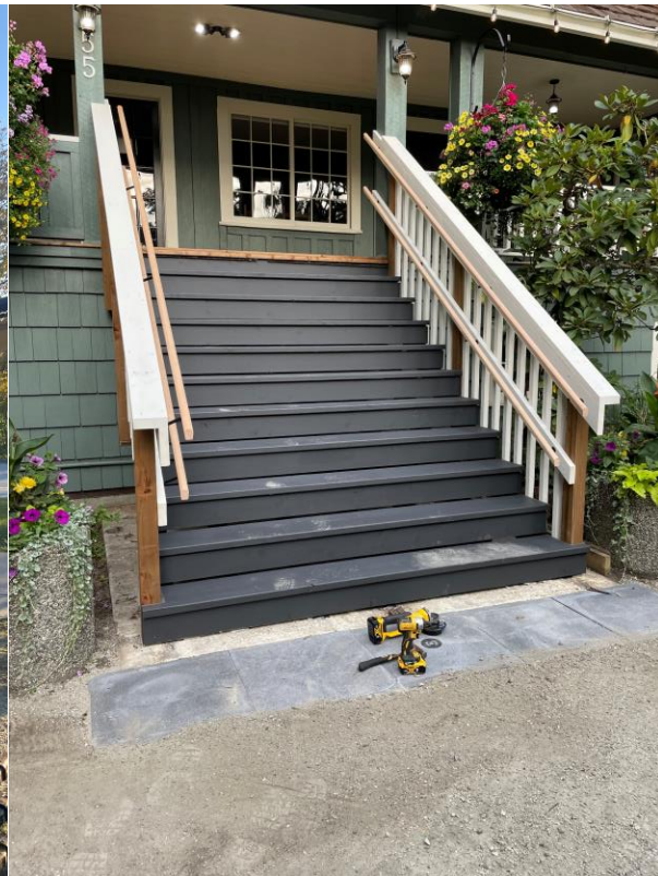
New staircase installed at Rockwood Lodge
