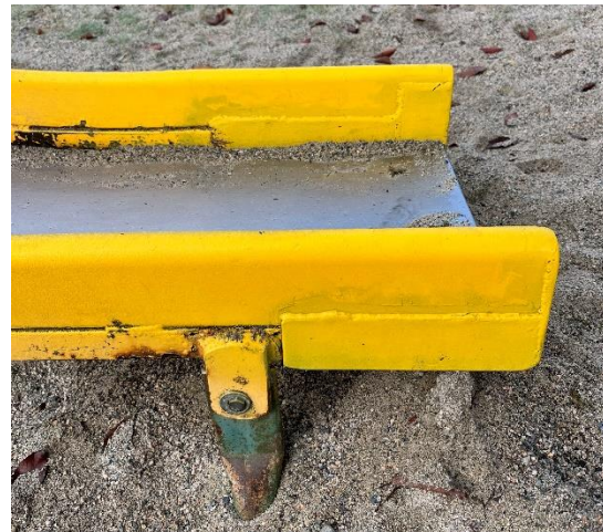
After: repairs & painting by Parks maintenance staff
