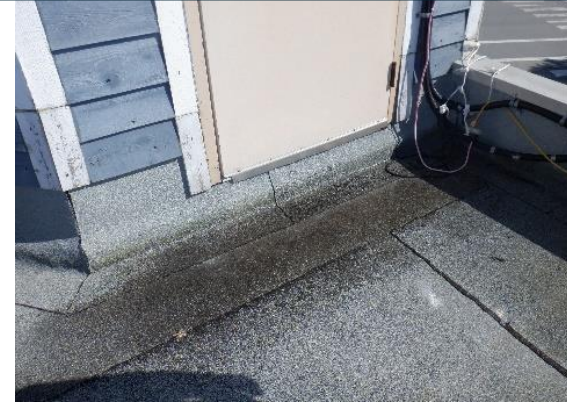
Roof Deficiency Photos of wear, voids and damage
