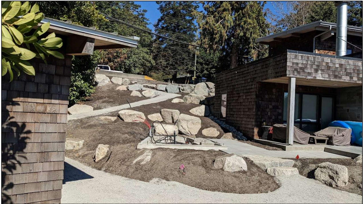
Figure 9. Opposite view of the RAA from Figure 8.
