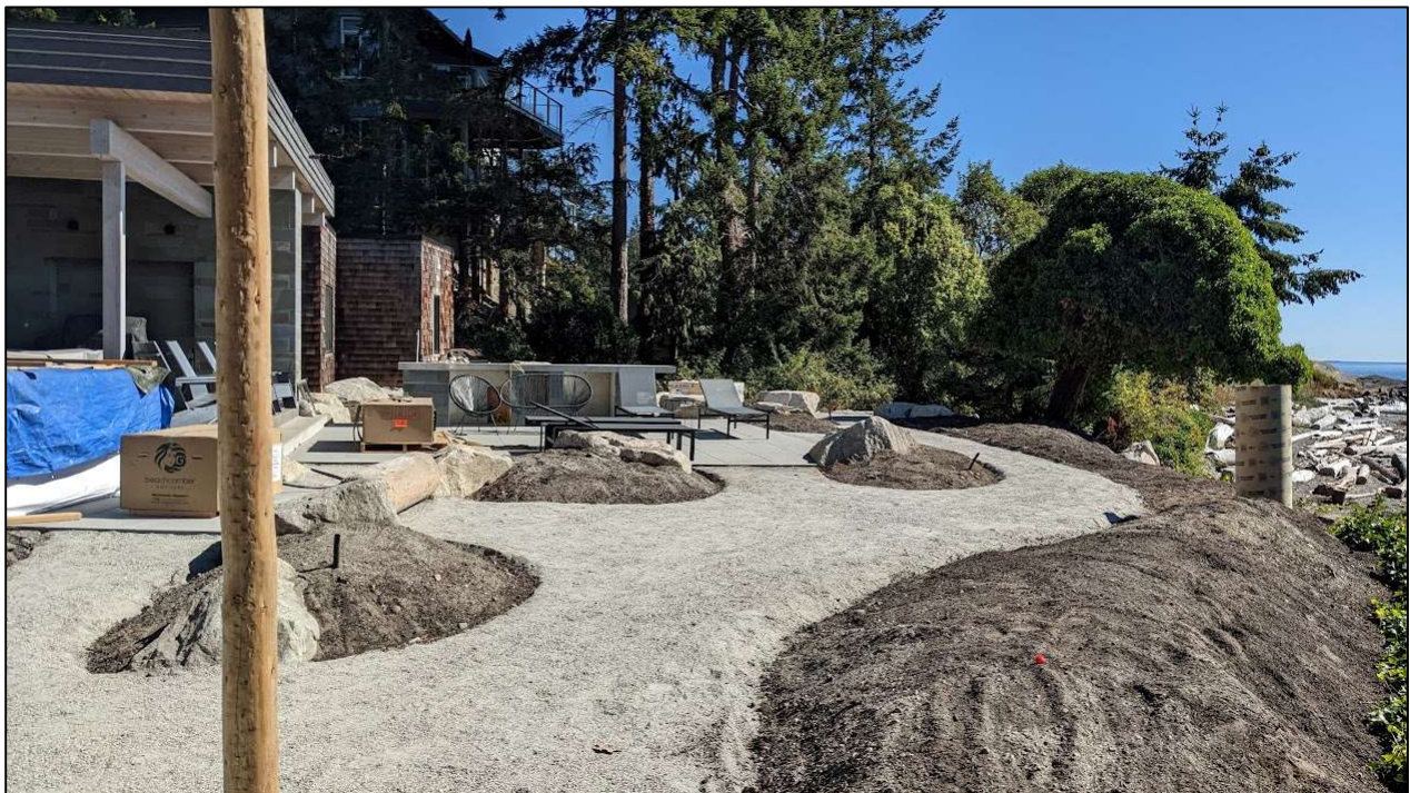
Figure 10. Viewing eastwards at the RAA and DPA-3.
